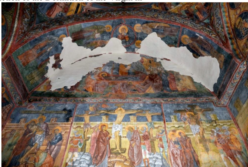
3. Holy Cross, Pătrăuți, western bay of the naos.
